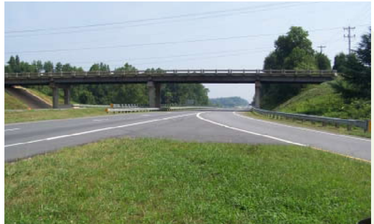
Existing Reedy Fork Parkway bridge over US 29 - North view.
