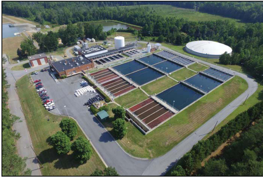
Townsend Water Treatment Plant
