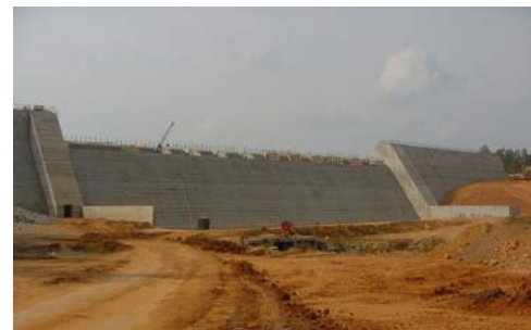
Randleman Dam under construction
