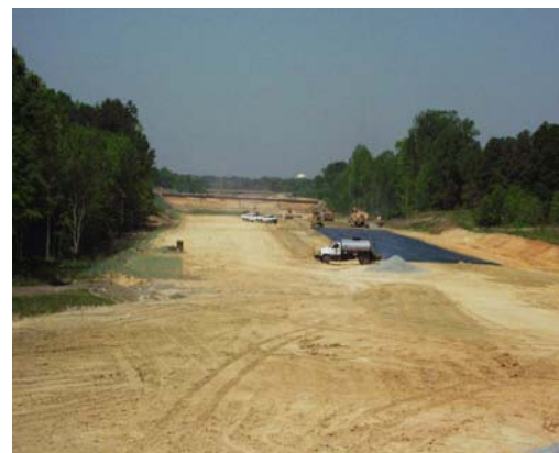
Urban Loop under construction
