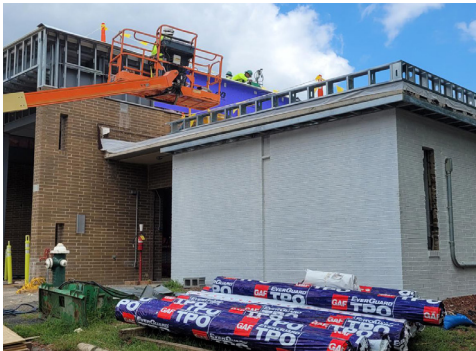
Fire Station Renovations
