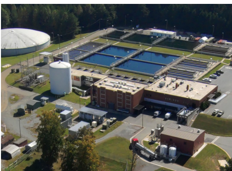
TZO Water Reclamation Facility
